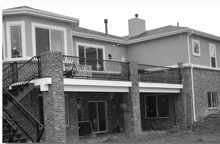
Full view of the back of the Castro home built in 2006 by Continental Partners, LLC, a company no longer in business but previously owned by Dominique Luzinski who now now operates Prime Builders, Inc. based in Centennial. He referred all questions about the Castro's complaints of his shoddy work, misuse of funds, use of sub-standard materials, plumbing leaks and lack of payment to subcontractors, to his attorney Art Pansing.
